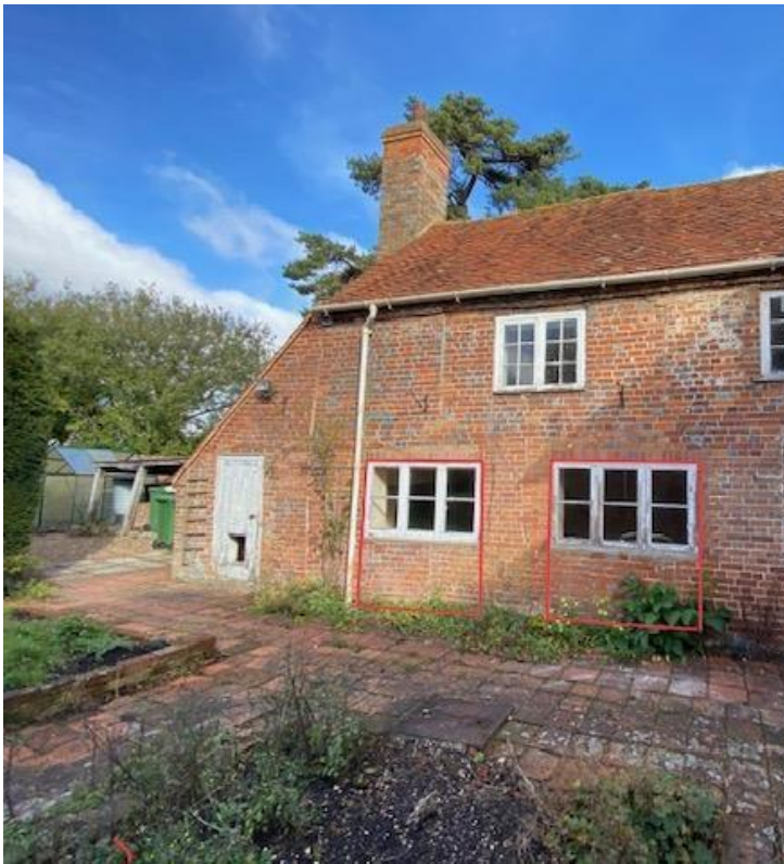
Figure 2: Location of new French doors on courtyard elevation
